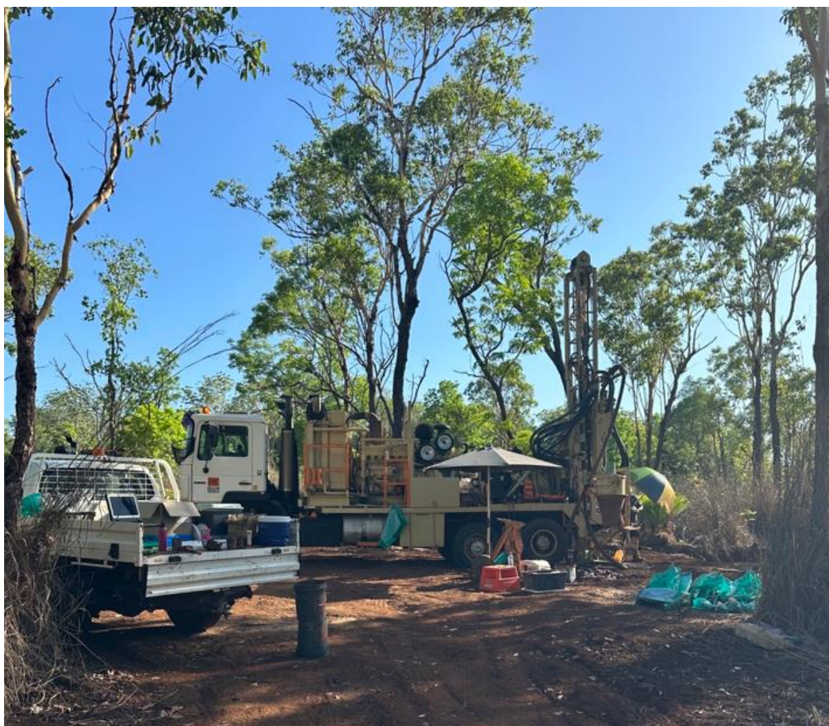
Figure 2: Commencement of Drilling at Yarram, MLN1163,
